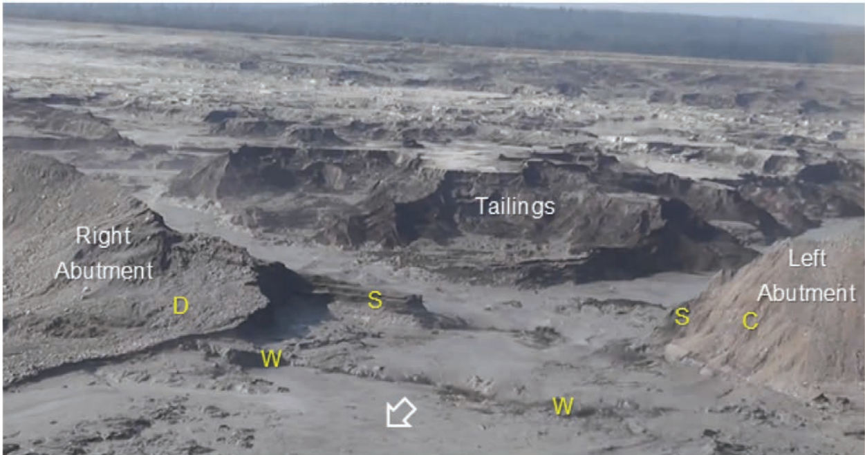
FIGURE 5.1.1: VIEW LOOKING UPSTREAM THROUGH THE BREACH (ARROW SHOWS DIRECTION OF OUTFLOW)
