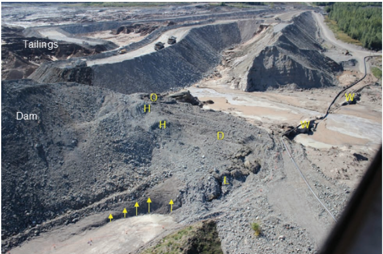
FIGURE 5.1.6: SLIDING-RELATED FEATURES AT RIGHT ABUTMENT (SEPT. 4, 2014 PHOTO)
