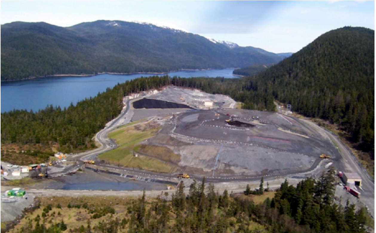
FIGURE 9.1.1 FILTERED TAILINGS FACILITY, GREENS CREEK, ALASKA
